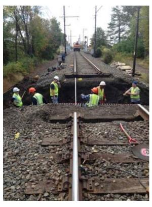
Villanova University partnered with SEPTA to install some pipes as a test installation underneath one of their lines; SEPTA and NCHRP covered the installation costs, materials for the project were donated by industry
